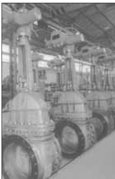
Gate Valves in stainless equipped with electric actuator
